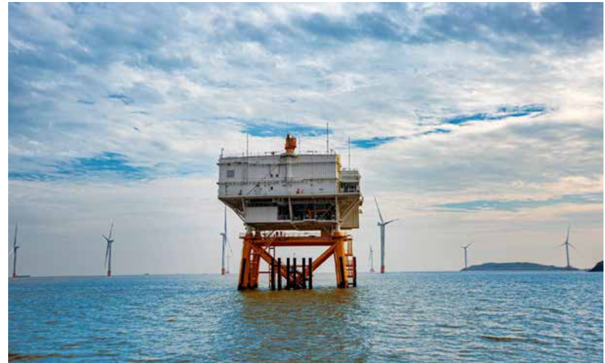
Zhoushan Offshore Wind Power Project
