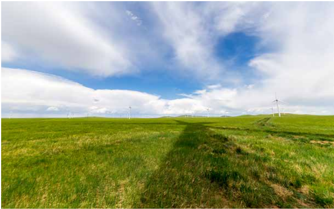
Inner Mongolia Onshore Wind Power Project
